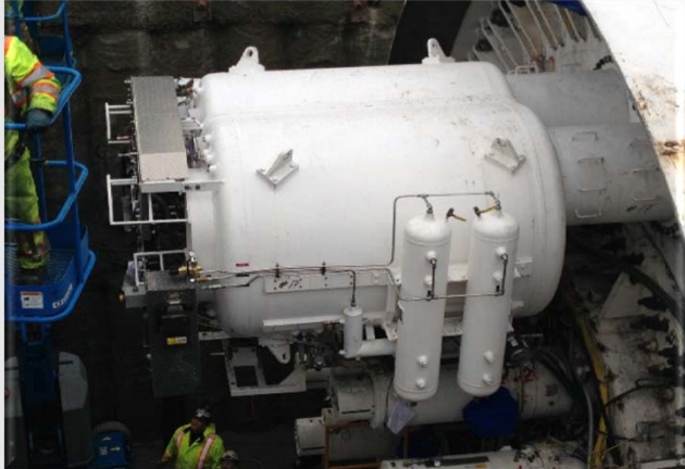
Typical Twin Air Lock on TBM
