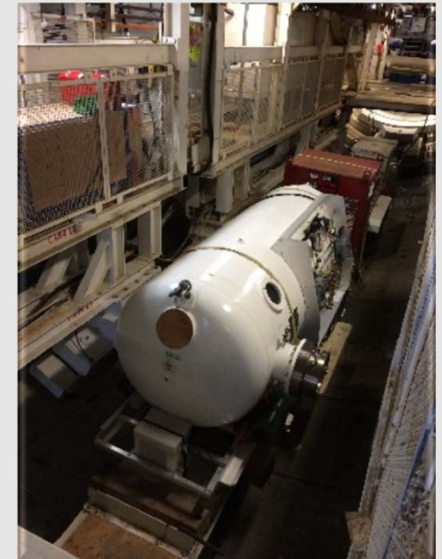
Transfer Lock in Tunnel
