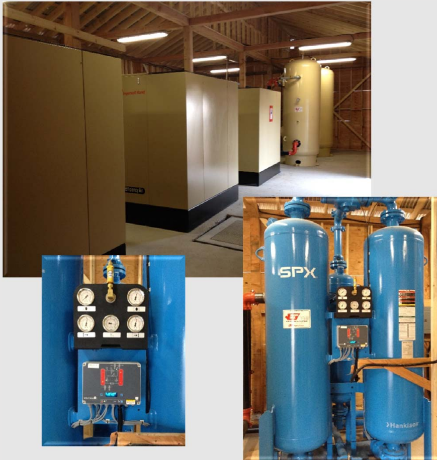
TBM Compressor Plant & Filtration
